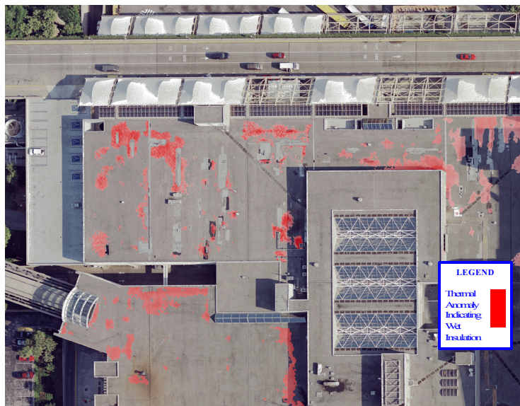
INFRARED2K Report: Section 1 Main Terminal
