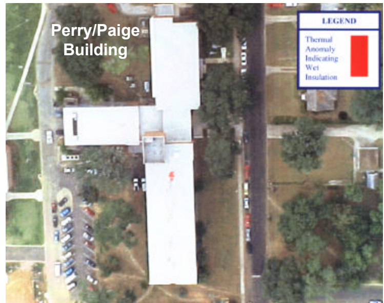
Inspection of a new roof exposes a small problem which can be corrected at minimal expense by the installing contractor.
