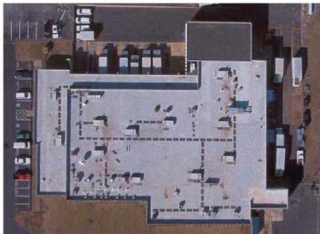
1) A daytime flyover in a helicopter to take a picture of the roof.
